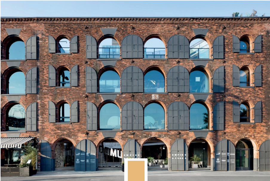
▼ Empire Stores by STUDIO V Architecture, a great example of adaptive reuse
