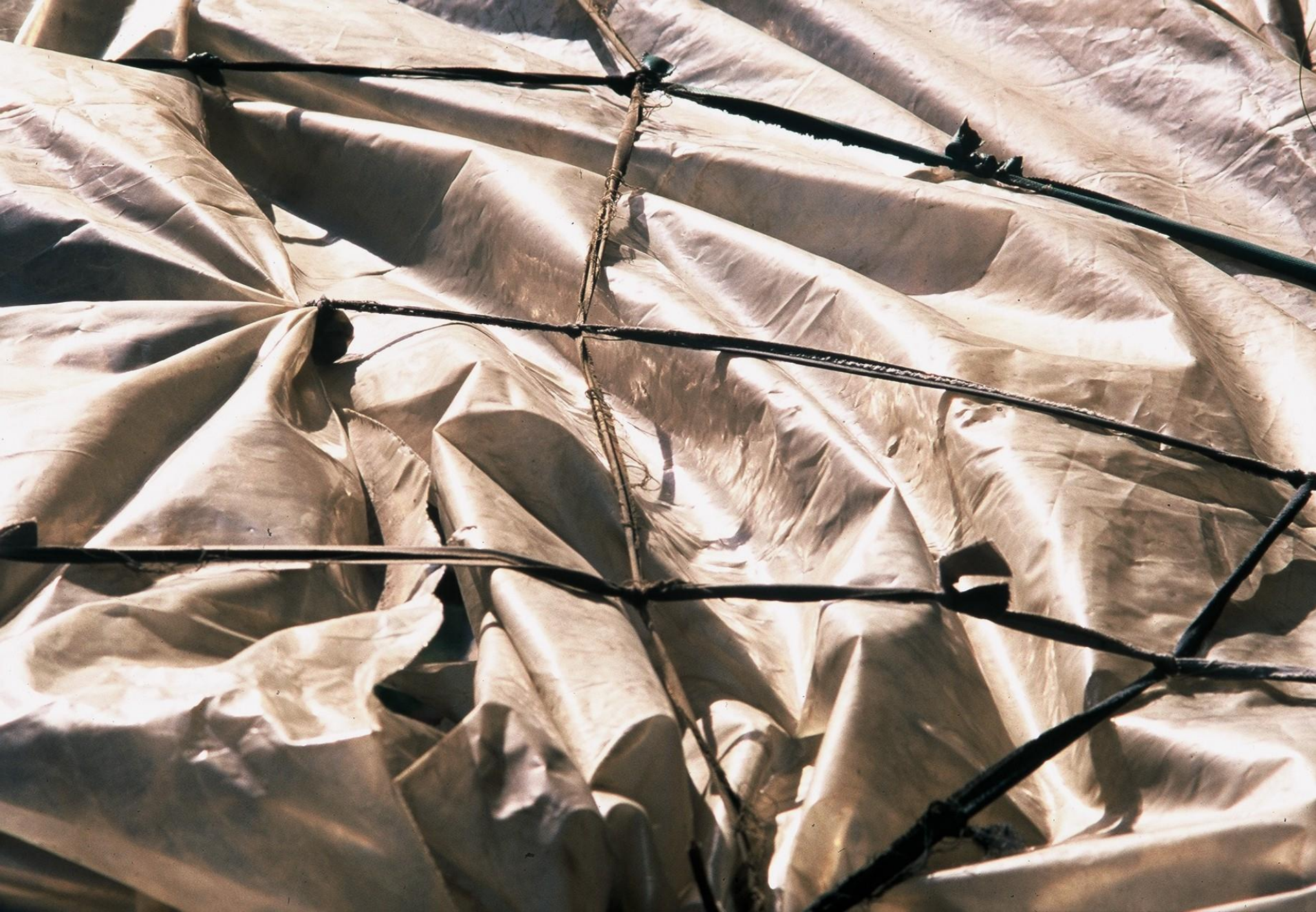
Roofs of houses were made like this from recycled plastic and rubber bands cut from old inner tyre tubes
